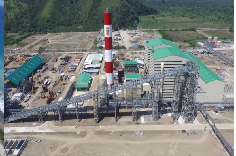
LIMAY 2X150MW POWER PLANT
