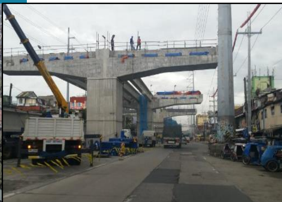
Ongoing works on Section 3
