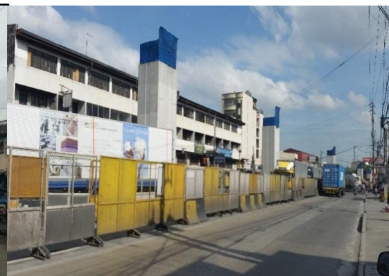
Ongoing works on Section 4
