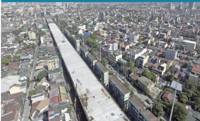
Ongoing works on Section 1
