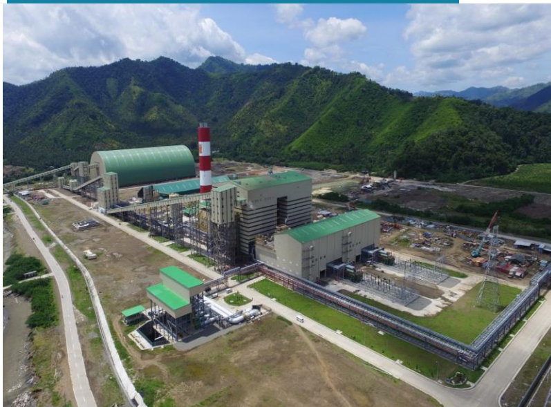
MALITA 2X150MW POWER PLANT
