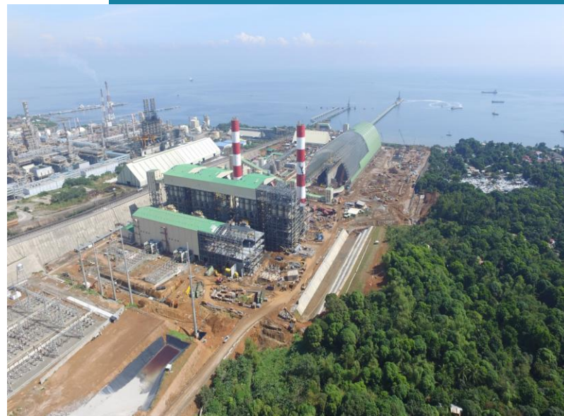
LIMAY 4X150MW POWER PLANT
