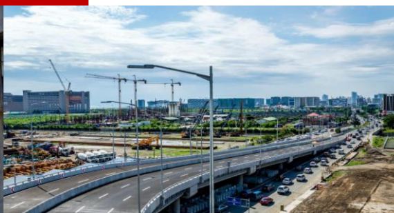
Completed ramps from Macapagal Ave. (Ramps 15-16)
