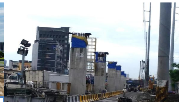
Ongoing works on Section 1
