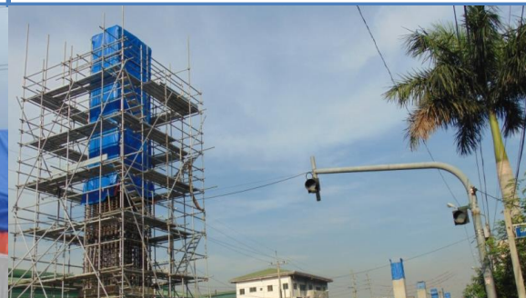
Ongoing works on Section 4
