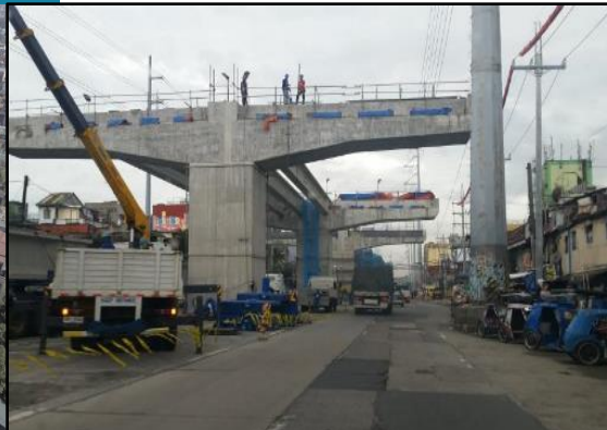
Ongoing works on Section 3
