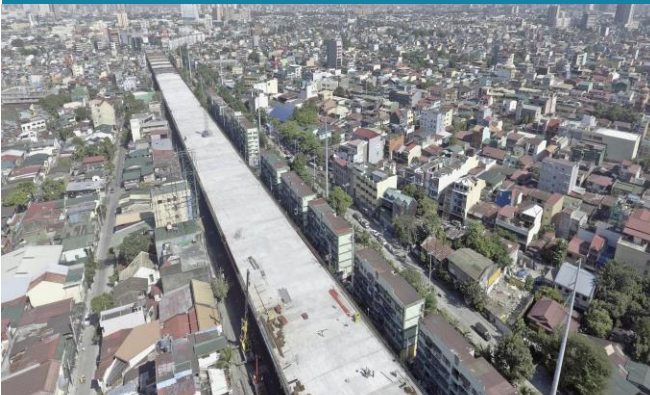
Ongoing works on Section 1
