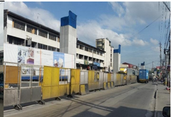
Ongoing works on Section 4
