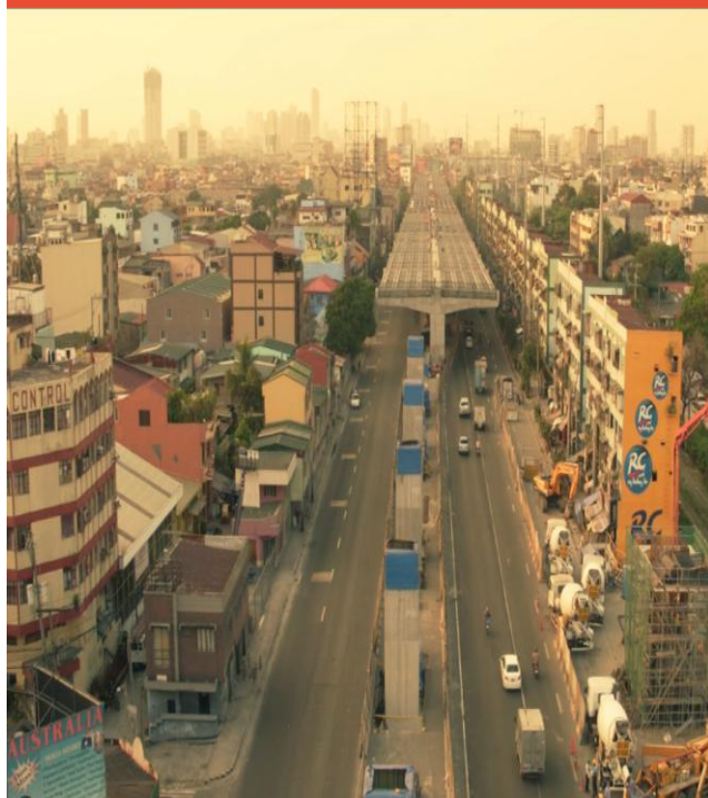
Ongoing works on Section 3
